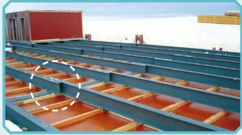
The station was constructed by securing the structural steelwork to the frame with Girder Clamps, forming a cross-girder base to support the accommodation block.
