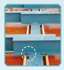
"Lindapter's product has performed admirably for us. With the foundations being 150m thick floating ice, flexure of the structure was a major issue which the Lindapter fixing system was designed to accommodate."
