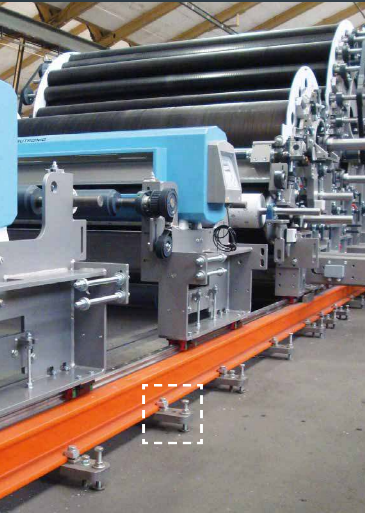
Photo shows a textile machine building production line, as the machines are built, they move along a rail which is attached to a steel beam. Lindapter clamps were used to connect the beam to the adjustable levelling strip assembly anchored into the concrete floor.
